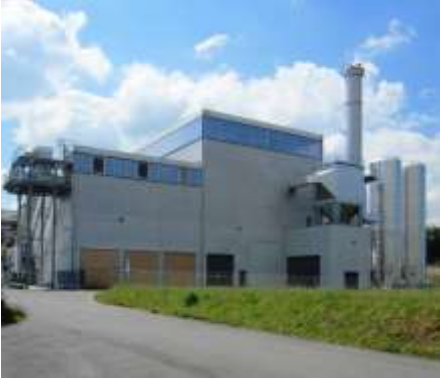
Image 1: The biomass CHP plant in Pratteln: sustainable, renewable and emission-free.
